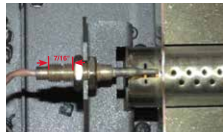
Diagram 4 Correct thermocouple placement
