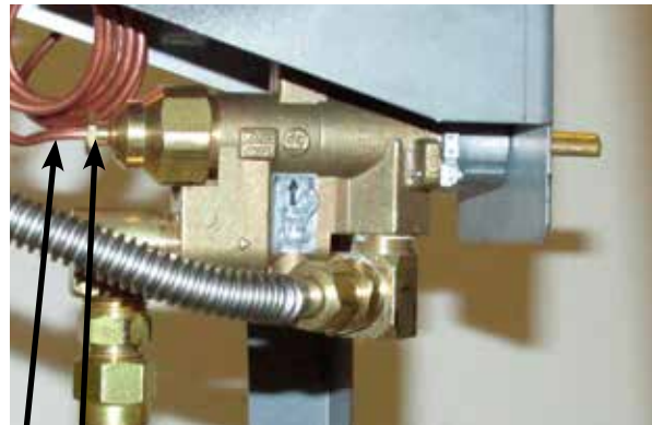
Diagram 3 Loosen nut to remove thermocouple
